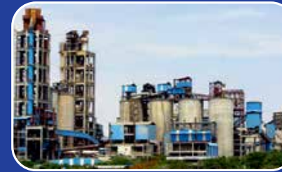
CEMENT PLANT MUKTYALA
